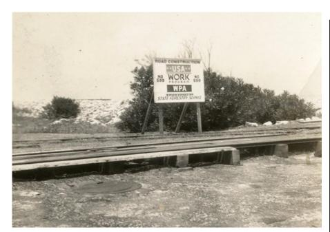
These pictures give you an idea of the manual labor which was involved in the construction of the highway. The cut and fill was accomplished with shovels and wheel barrows, which had iron wheels, would sink into the sand, and had to be moved on plank paths. There was no base. The surface was asphalt and sand, mixed in place. In hot weather a load would sink into the surface.
